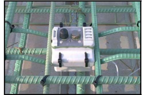
The ECI-2 During Installation in a Bridge Deck
